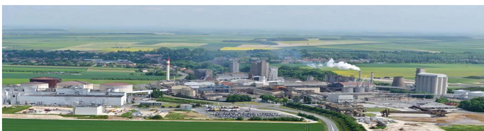
At the heart of the Biorefinery Platform of Pomacle-Bazancourt near Reims (F) 18
